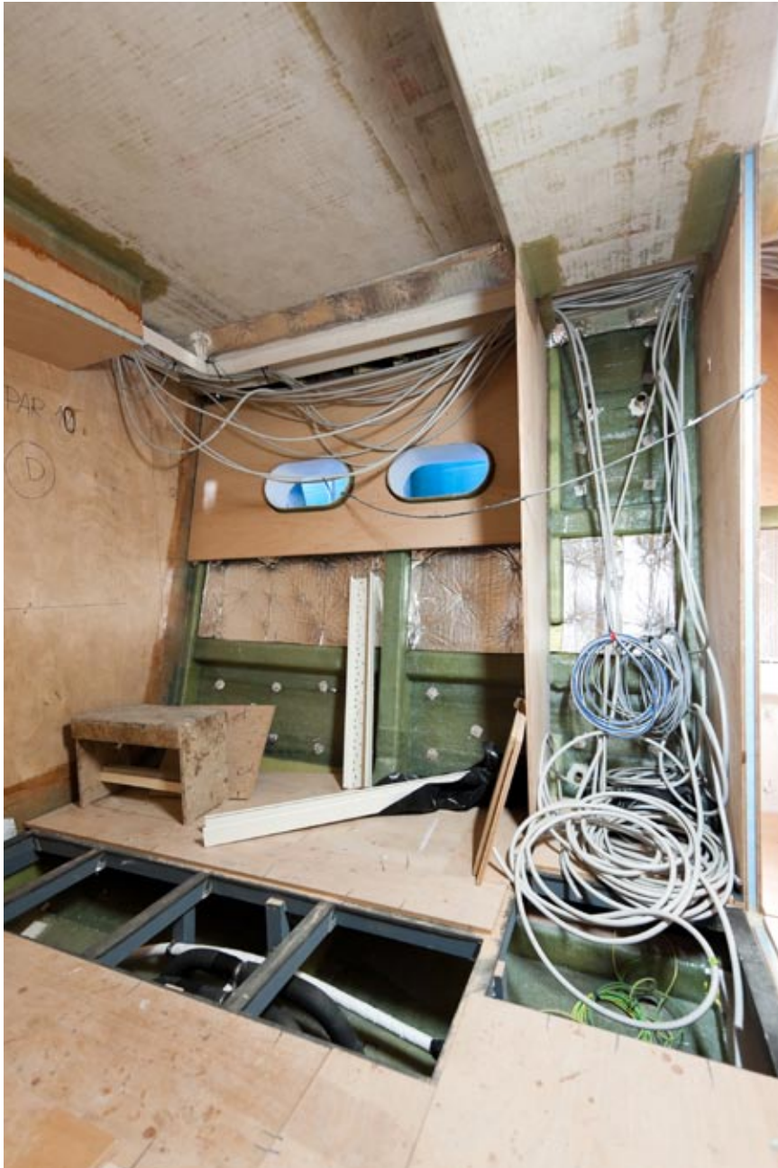
Cabina Armatore (in costruzione) / Shipowner cabin (under construction)
