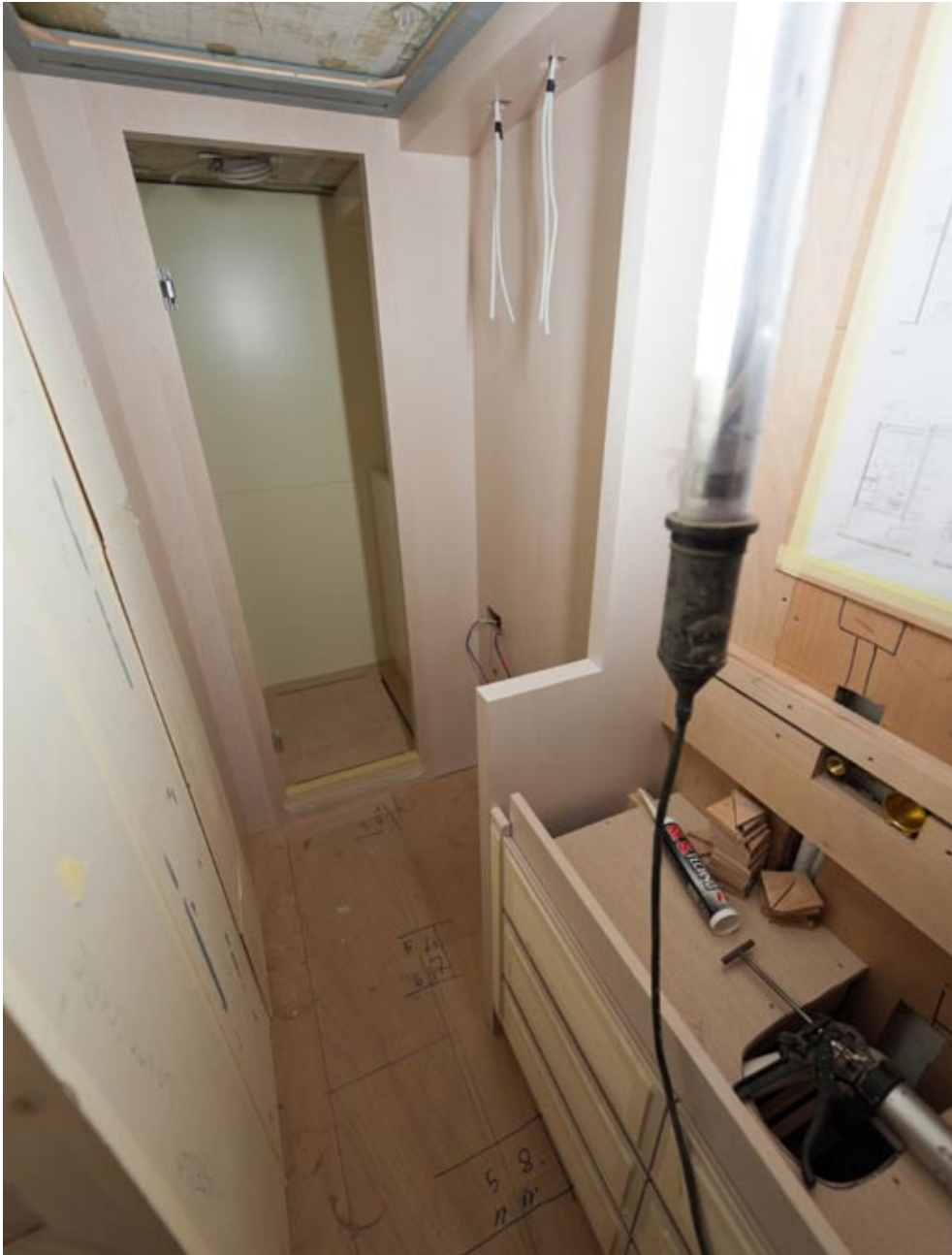
Bagno cabina Armatore (in costruzione) / Shipowner cabin bathroom (under construction)
